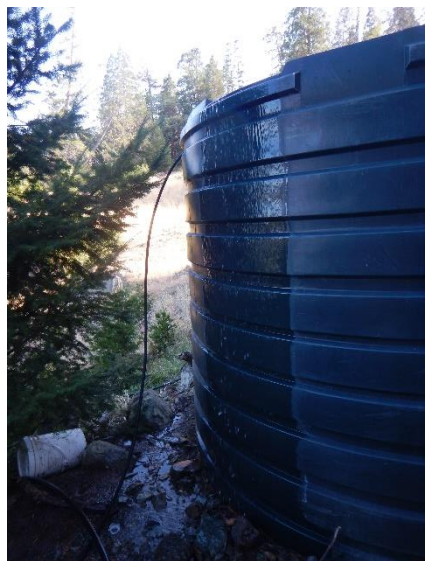
Photo 33: Storage tank, associated with T2-4, actively leaking from the top of the tank, showing overflow valves either not installed, or functioning properly.
